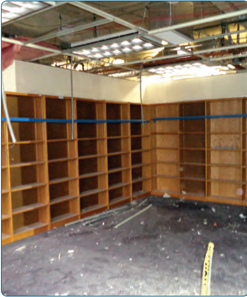
Above: The new EPA library includes most of the furniture, fixtures, and equipment from the old library. All the original stacks, carrels, and seating were reused.
